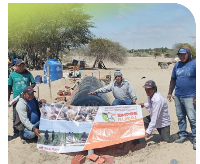
➤ Installation of 02 Biodigesters with gas holders and industrial kitchens in the Sechura desert areas such as Chutuque and El Barco, which will allow Biol to be obtained for their crops and biogas for the operation of industrial kitchens.
